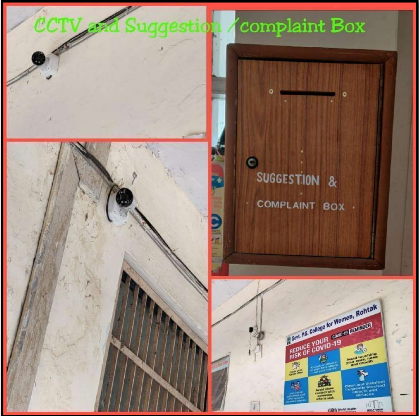
CCTV and Suggestion / Complaint Box
